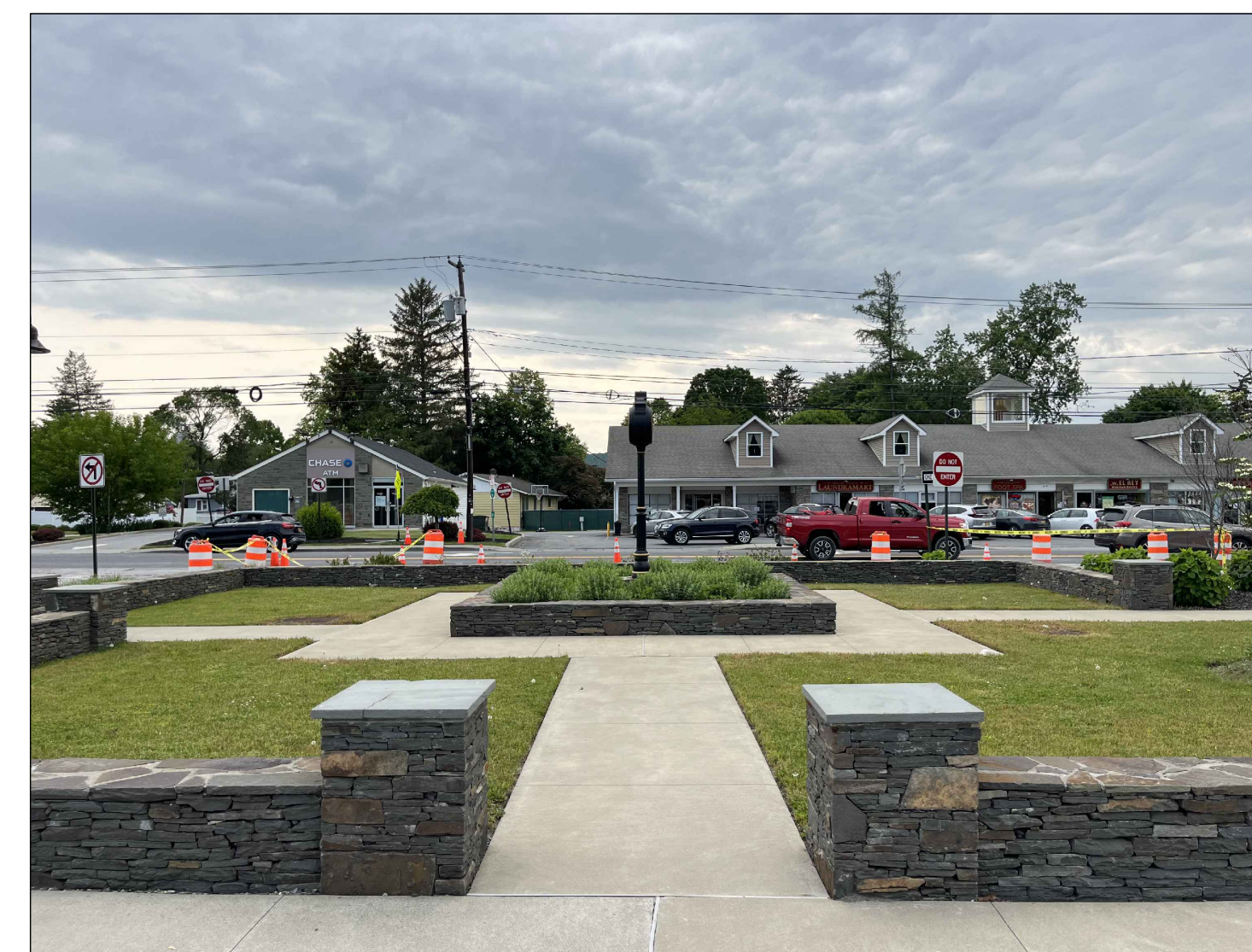
All new and proposed walls and columns to match the existing wall and column style
