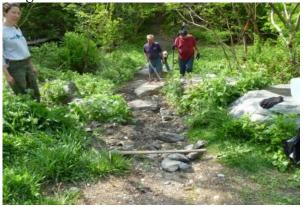
While on site, efforts were also made to clean out and armor all of the culverts in order to prevent flooding. We also created drainage swales along the trail to prevent erosion. We did a thorough cleaning of the site and removed litter and some old tires and a couch that had been illegally dumped on site.
